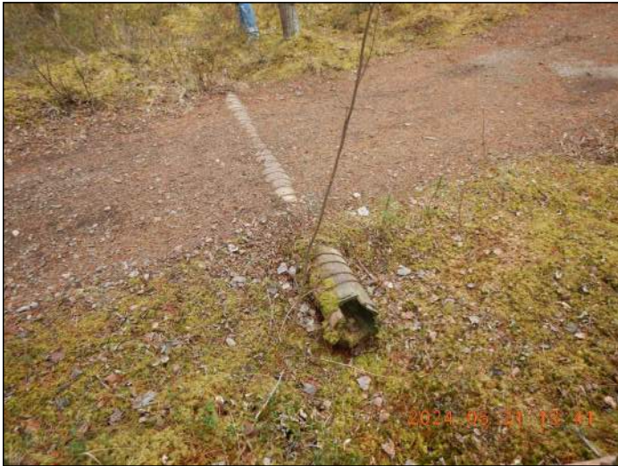
EXISTING WOOD STAVE CULVERT
