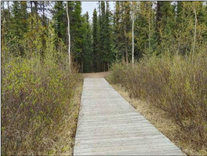
TYPICAL EXISTING TIMBER BOARDWALK
